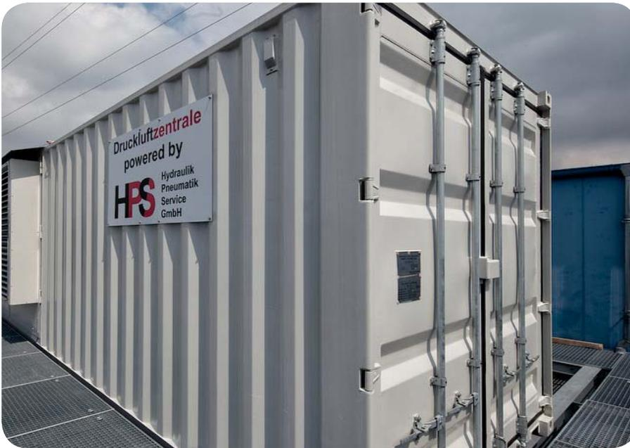
The container compressed air station is optimally located at a central point on the roof of a production building.
