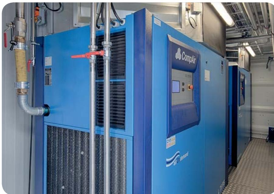
**Three 75 kW regulated speed compressors generate the compressed air that the GKD factory needs.**
