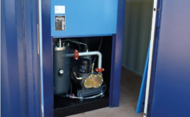
The key issue was that the compressor housing had been constructed around the machine. As a result, it would not be able to accommodate a new system without extensive structural work.
